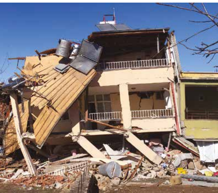
Effects and soft-story damage to non-seismic resistant buildings.
